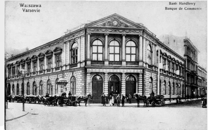
Historical Head Office of the Bank, Warsaw, 7/9 Traugutta Street
